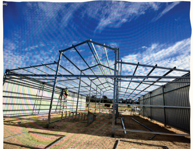
Building Piggy Paradise, a purpose built home for our pigs.
